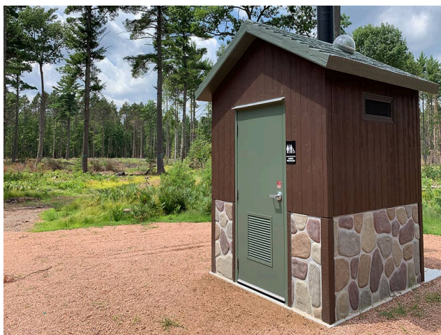
AFTER: New pit toilet building
